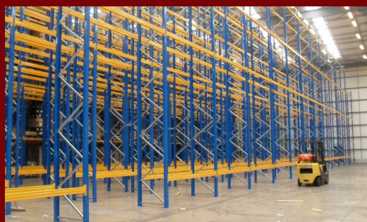
The start of the racking extension
